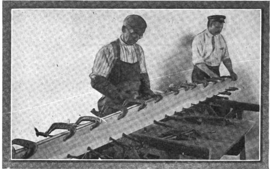
Fig. 2—Clamping the three laminations together after they have been glued
